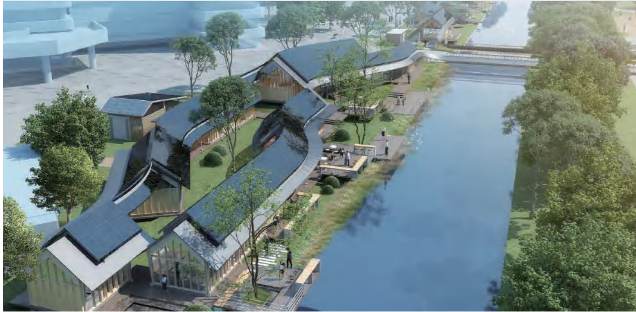
Yancheng, Jiangsu | Xifuhe Green Low-Carbon Sci-Tech Park Zero-Carbon Station
