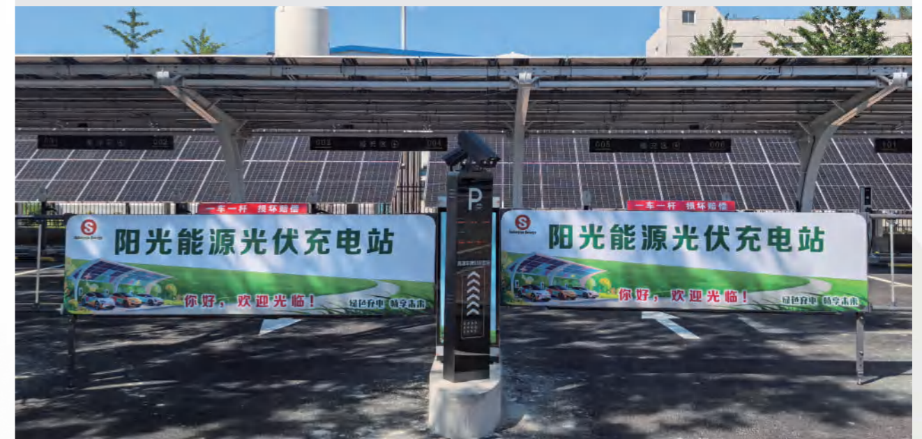
Jinzhou, Liaoning | Solargiga Integrated PV, Storage & Charging Station
