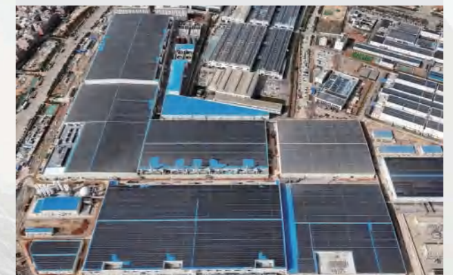
Qujing, Yunnan (2023) 32.41MW Distributed Power Station
